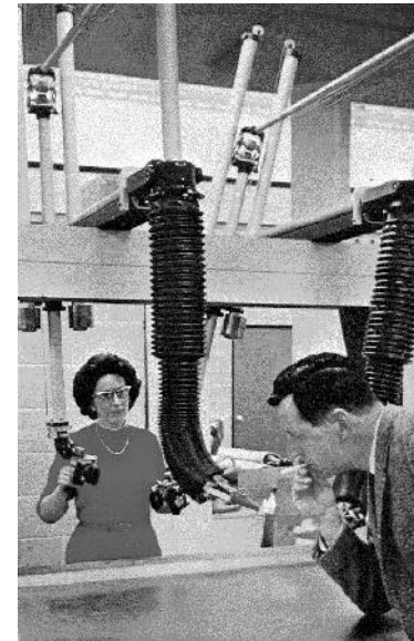
Early teleoperator system with mechanical kinesthetic force feedback.
